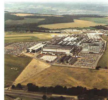
Aerial view of Airport Works, Rochester
