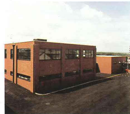
Falcon Building at Rochester has specially stabilised foundations for high precision manufacture.
