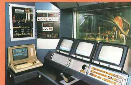
Testing gas turbines automatically, using this computerised system, makes testing quicker and more reliable, prolongs engine life and saves fuel. The system has been supplied to four air forces.
