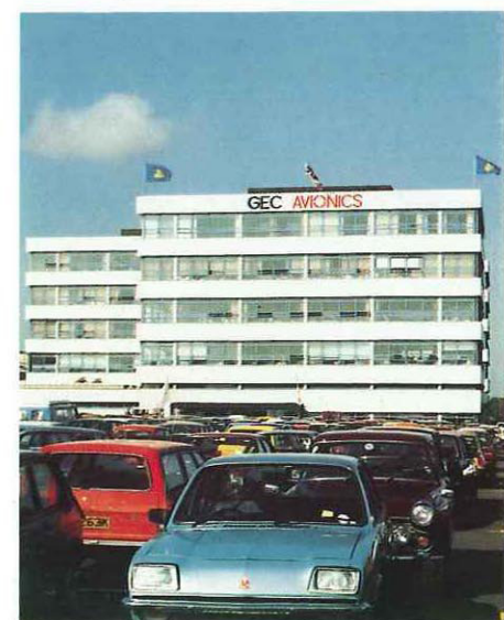
Towers Site, Airport Works, Rochester
