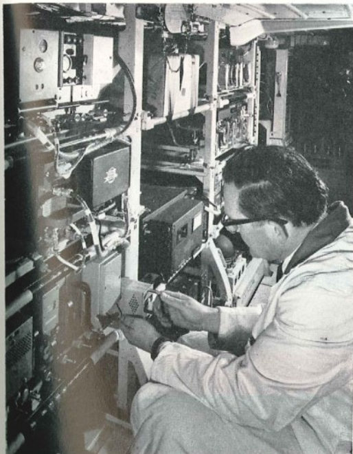
Maintenance contracts are undertaken by Heathrow Airport, London, Depot
