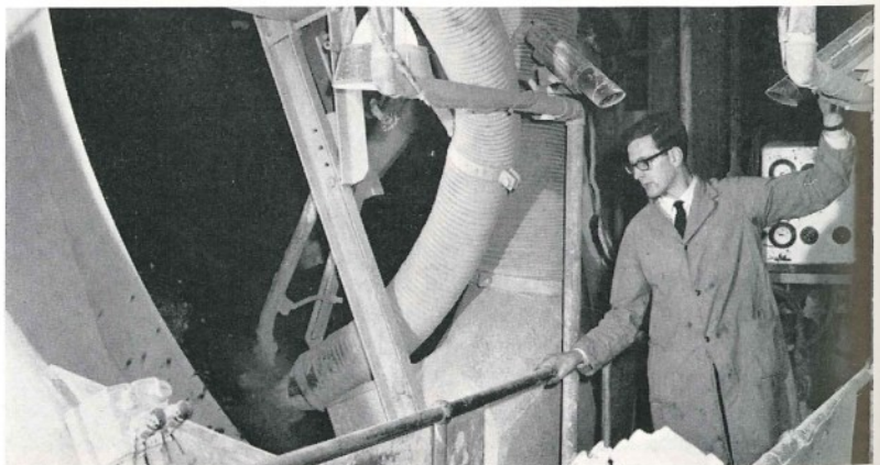
Cameras viewing the interiors of 'nodulizer' pans in a cement works
